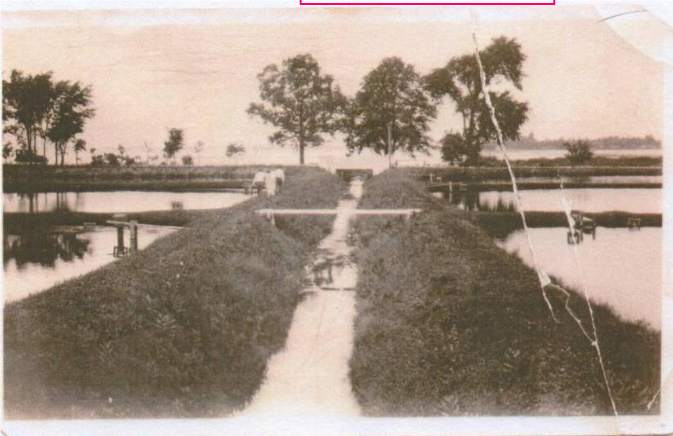
Old dam and channel 1914. Facing South.
