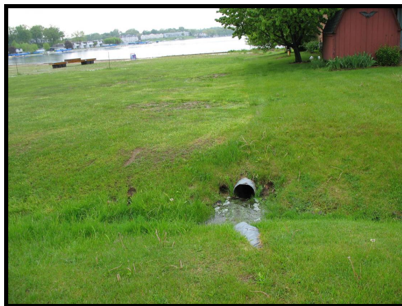
Figure 9.4b. Downstream of road.
