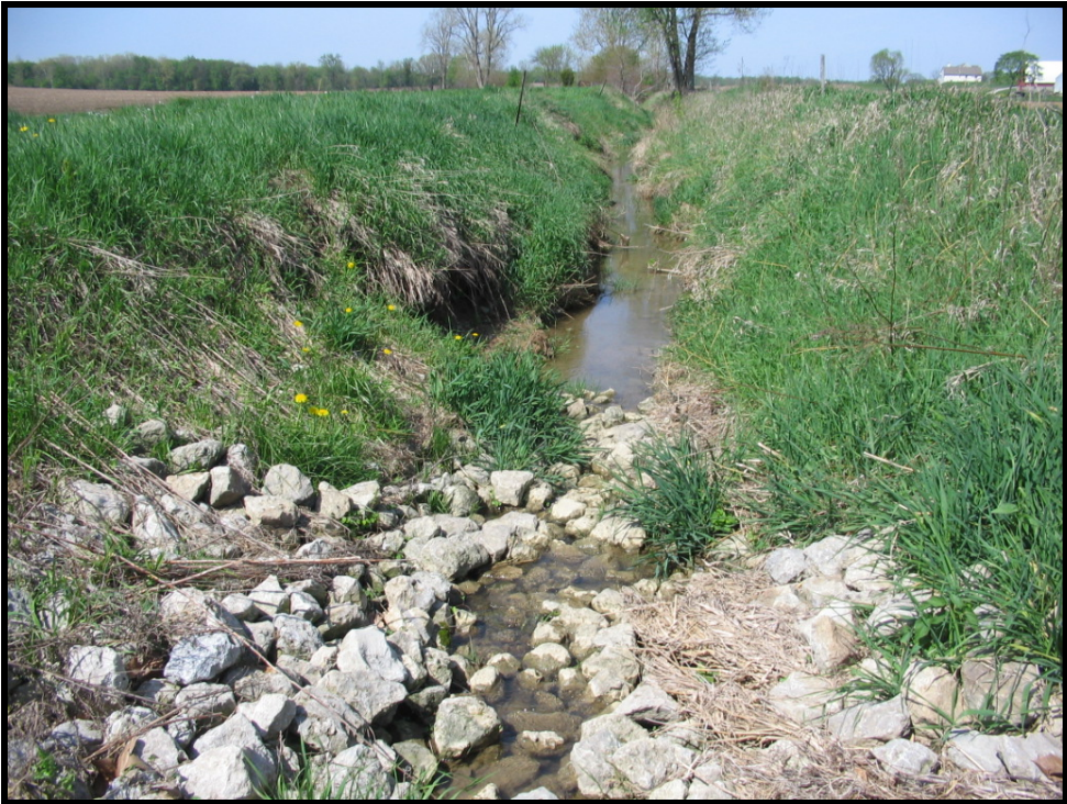
Grade control structure installed along Dillon Creek through the Watershed Land Treatment Program with the cooperation of the Noble County Surveyor's office.
