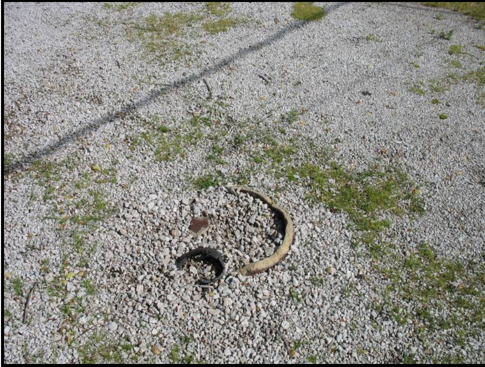
Figure 5.3. Gravel-filled storm drain.
