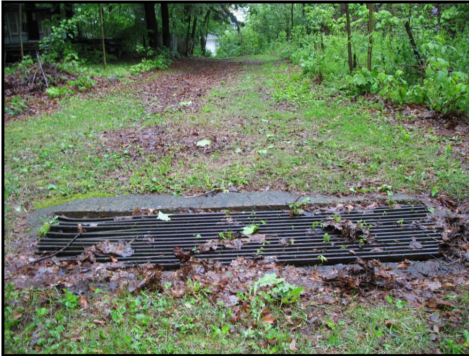
Figure 10.1. Metal grate covering 2x2 foot drain pipes.
