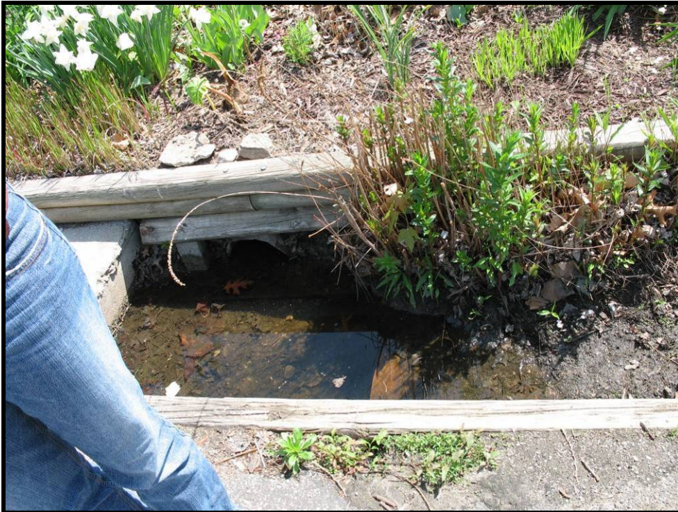
Figure 5.9. Storm drain draining road runoff into lake both directly and via the channel to the south.
