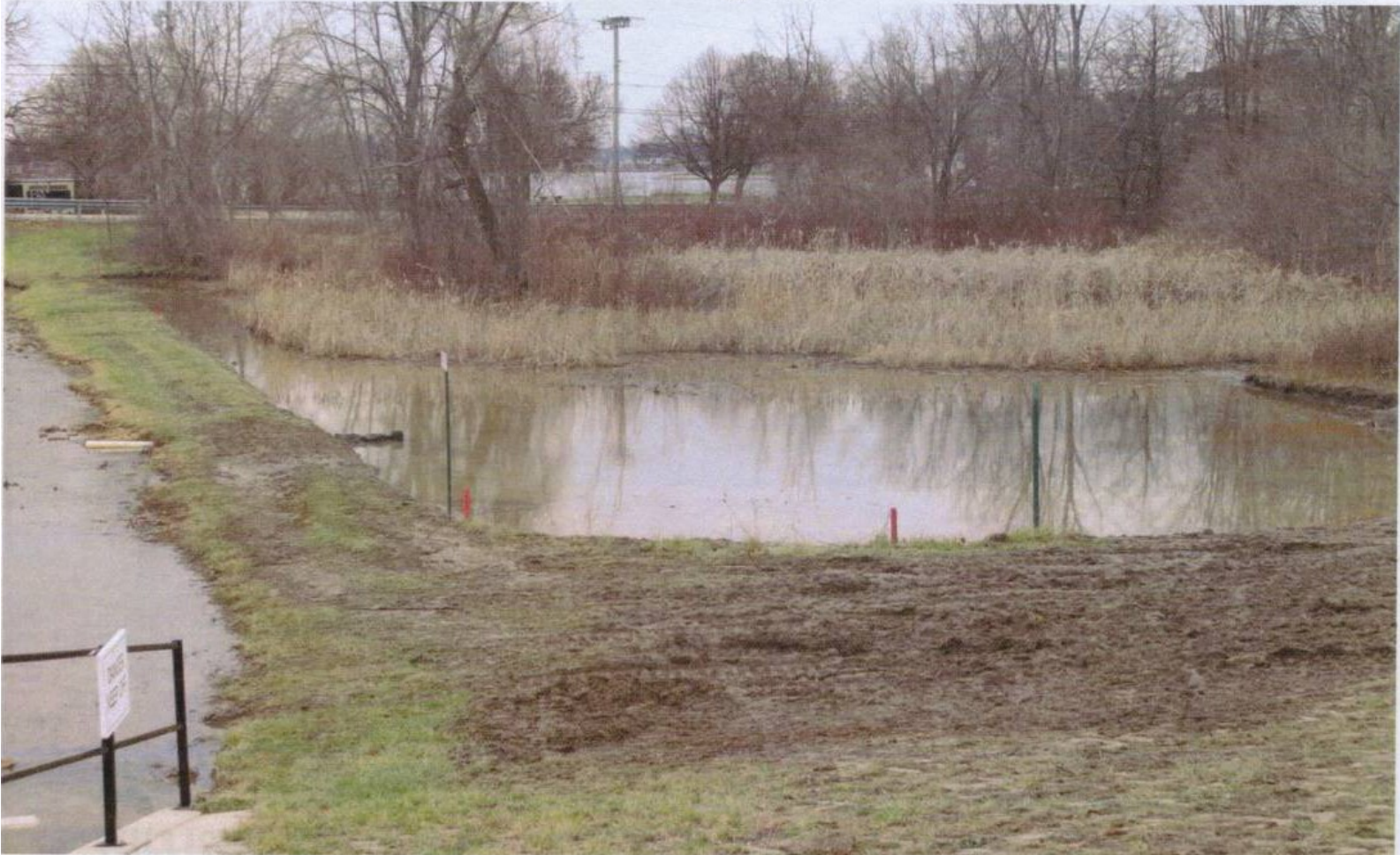
Photo Point 4: SITE Following Re-Grading Activities, 10 December 2014 View: Facing North
