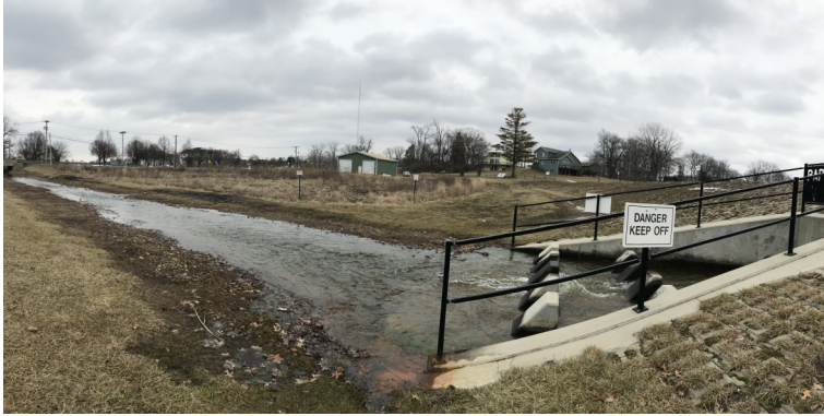
Standing on top of dam facing Hatchery Road
